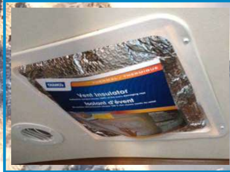
Thermal Insulated Bedroom Ceiling Vent
