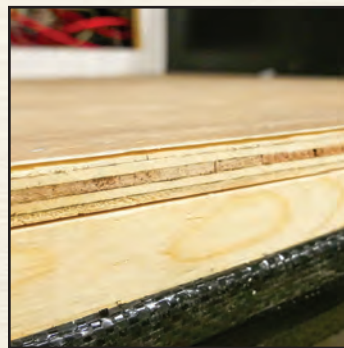
TONGUE & GROOVE PLYWOOD MAIN AND UPPER FLOORS
